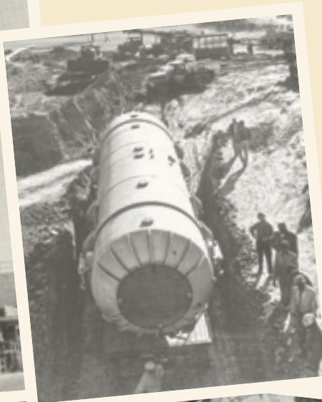
Clockwise from top left: The FSU Nuclear Research Building in 1960. The installation of the first EN tandem Van de Graaff accelerator in 1959. The EN tandem Van de Graaff accelerator being assembled at the lab in 1959. Nuclear physics student Kuick Lee and nuclear theorist Alex Green. Photos courtesy Florida Memory and FSU's Digital Research Repository.
